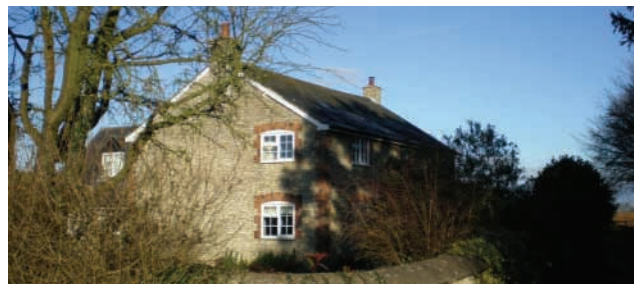
Larkwell, brick detailing in the limestone construction
