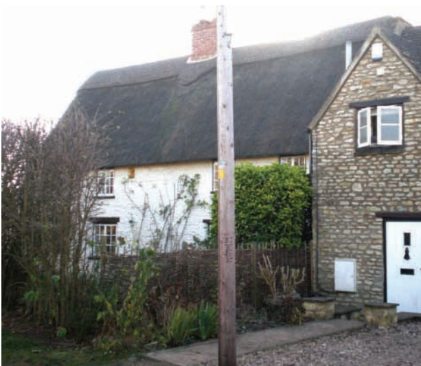
Vernacular thatched roofs have been largely replaced by slate and tile
